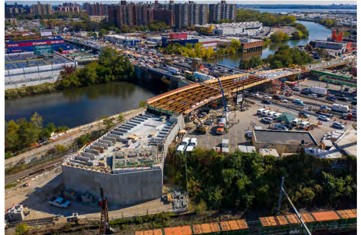
Aerial view of the construction of the "island"
