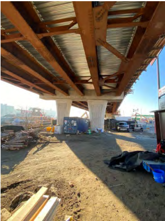
Integral Pier Construction
