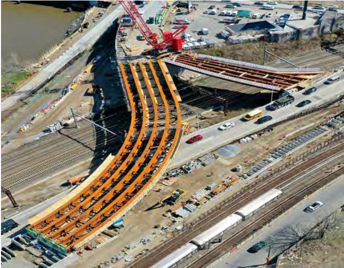
Construction of Ramps ES and SE over the NE corridor
