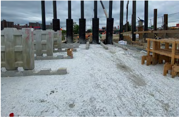
Lightweight Cellular Concrete Fill used in the retaining wall system
