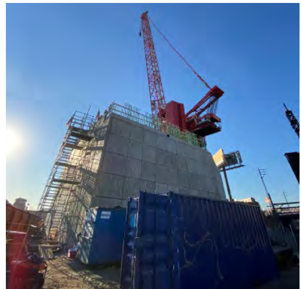
Manitowoc MLC-650 Crane on top of the Island
